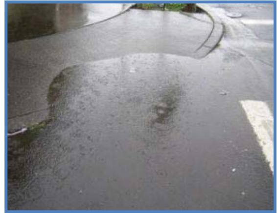
Drainage issues at a curb ramp downtown
